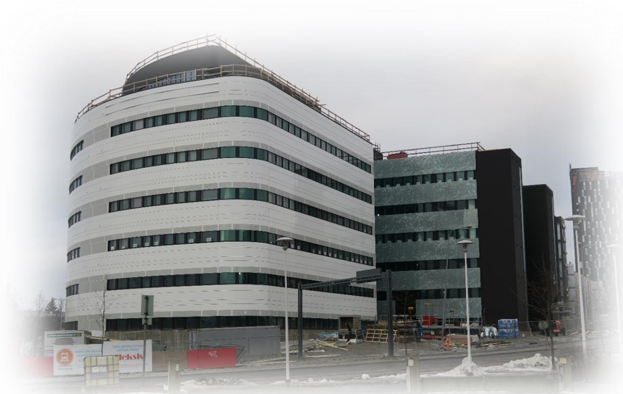
Yliopistonrinne CD building under construction in Tampere
